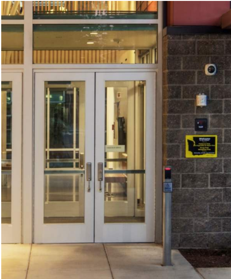
Figure 1 Main Entrance with controls requires screening at Main Office
