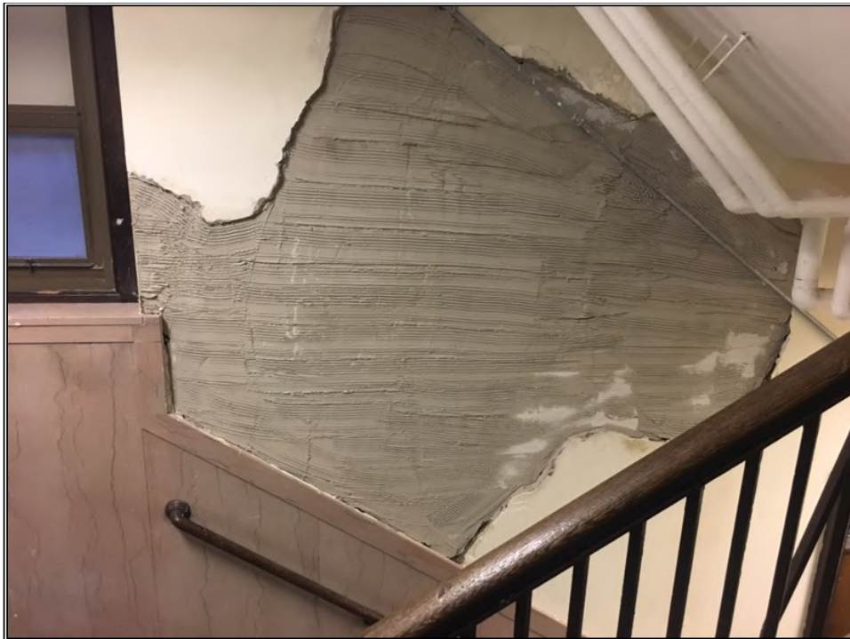
Photo 2: Plaster Repair on Damaged Wall
