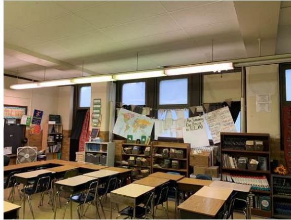
Typical Classroom Windows
