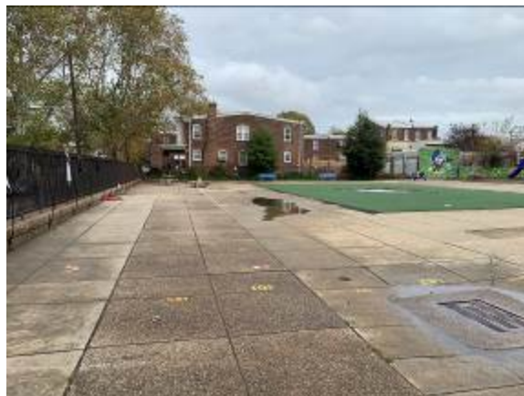
Concrete play surface
