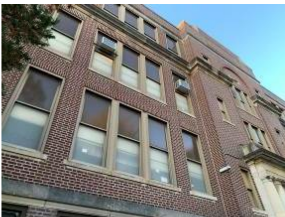
Northwest Upper Façade
