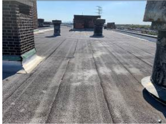
Typical Roof Condition
