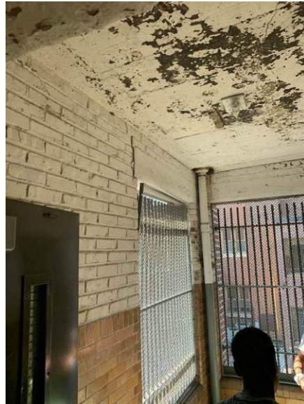
Exterior Egress Stairway
