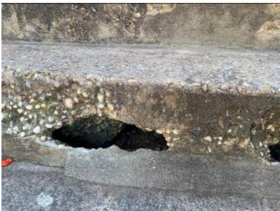
Concrete Stair Riser
