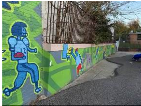
Residential side retaining wall
