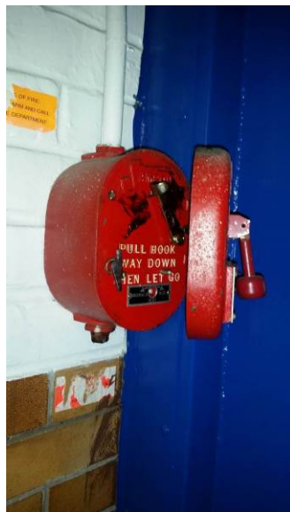
Typical Fire Alarm Device
