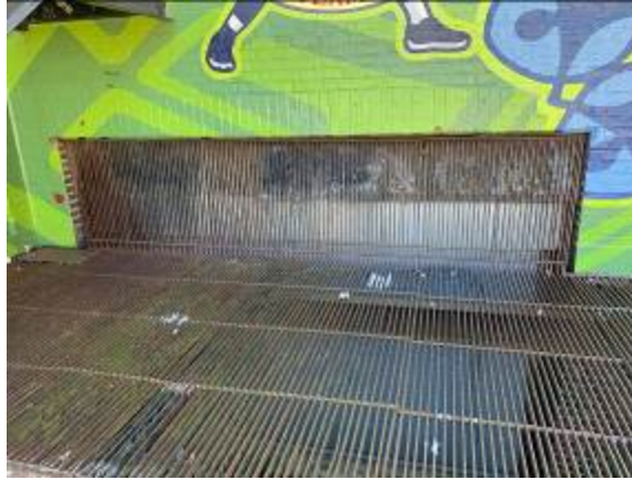
Rear Ventilation Opening and Lintel
