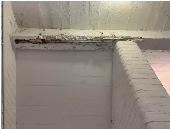
Exterior Egress Stairway
